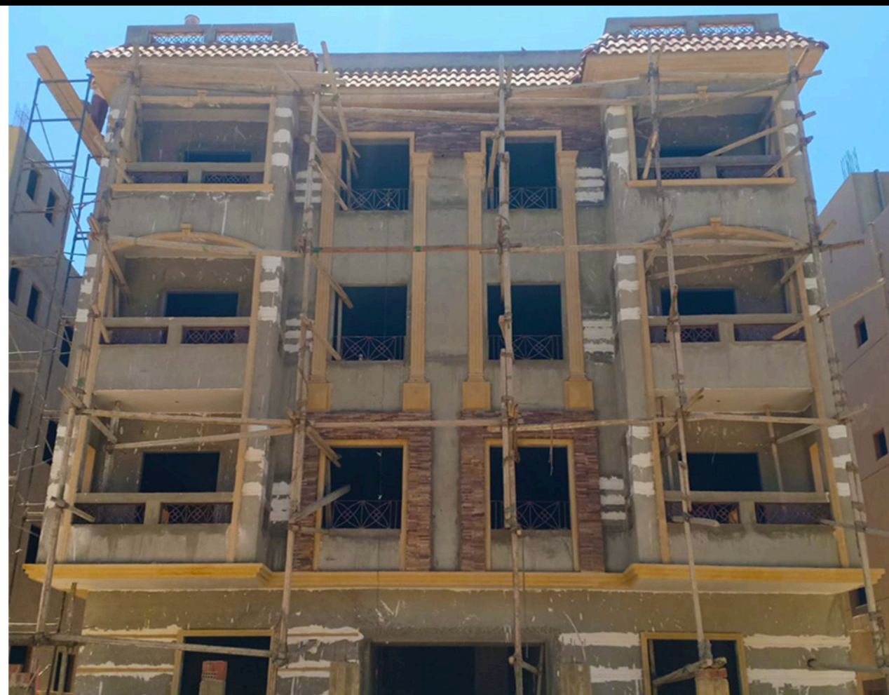
Facade works villa lotus 843
