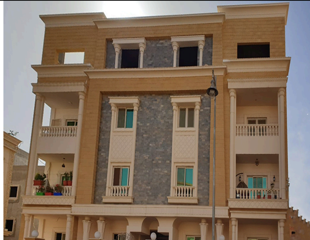
Facade Works villa 365 lotus
