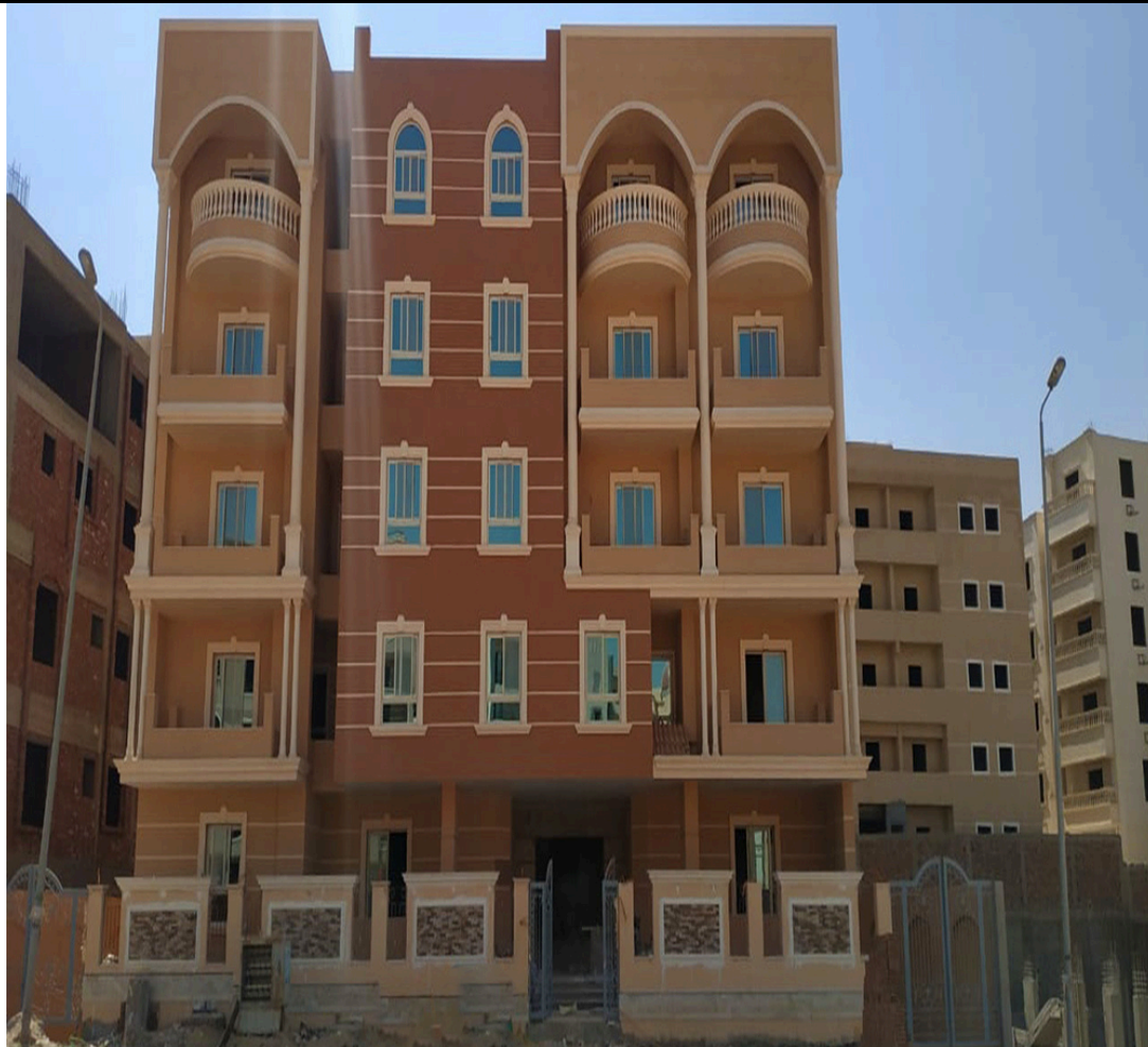
Facade works villa lotus 126
