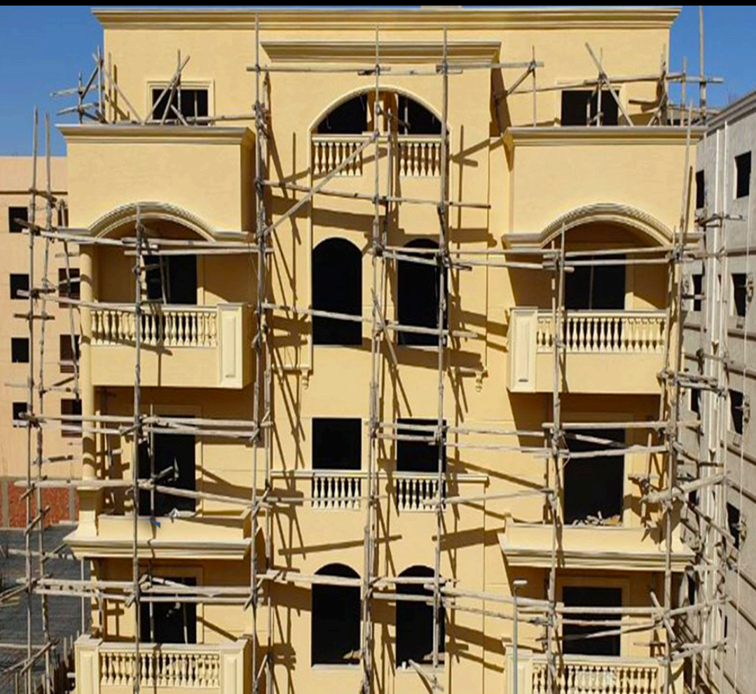
Facade works villa 228 alandalos
