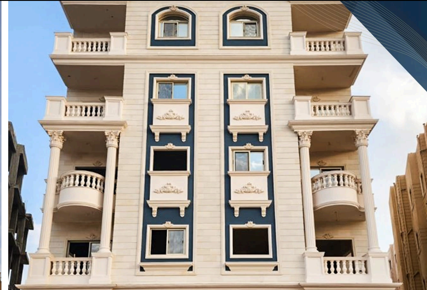
Facade Works at al andalos
