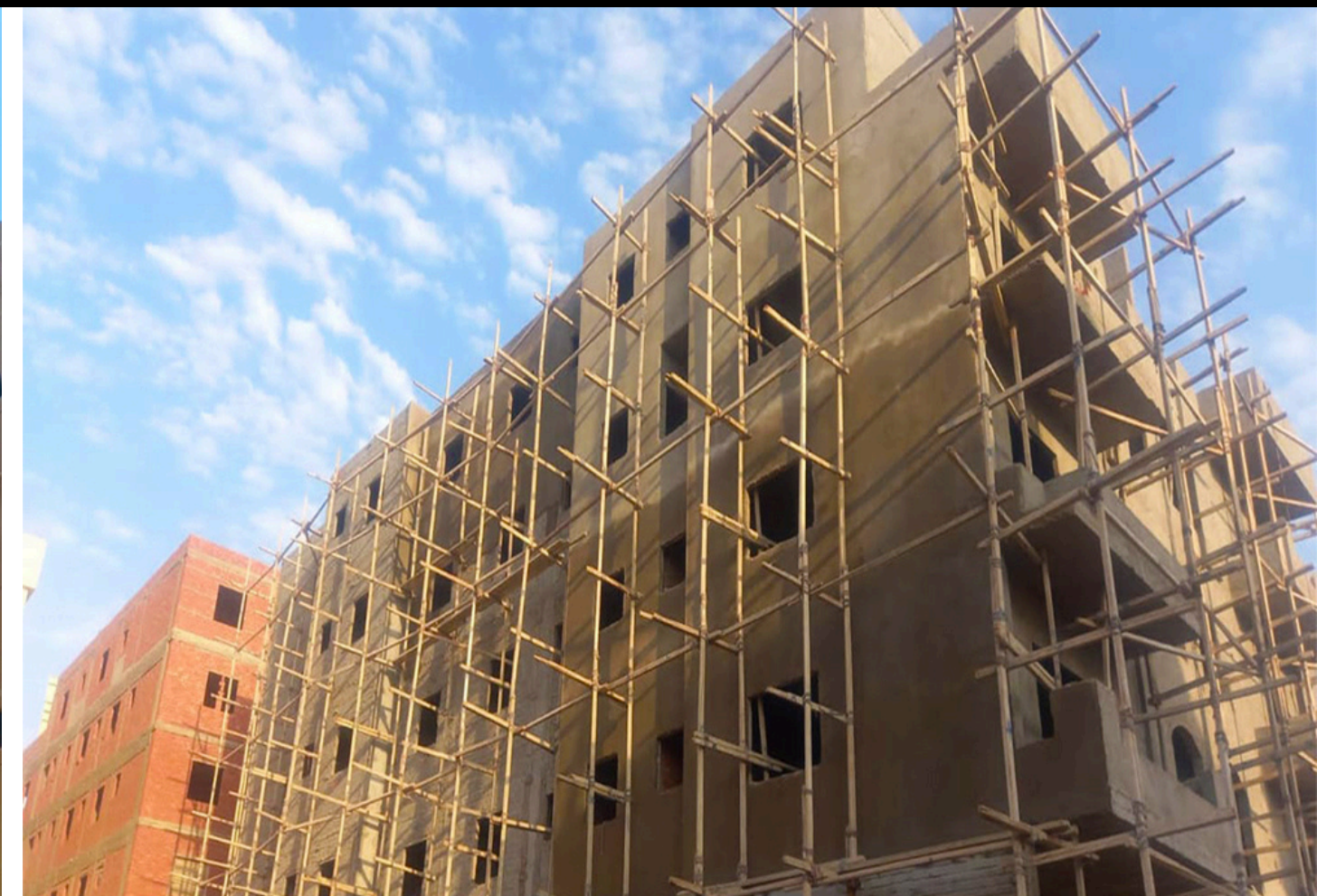
PLASTER Works villa 228 alandalos
